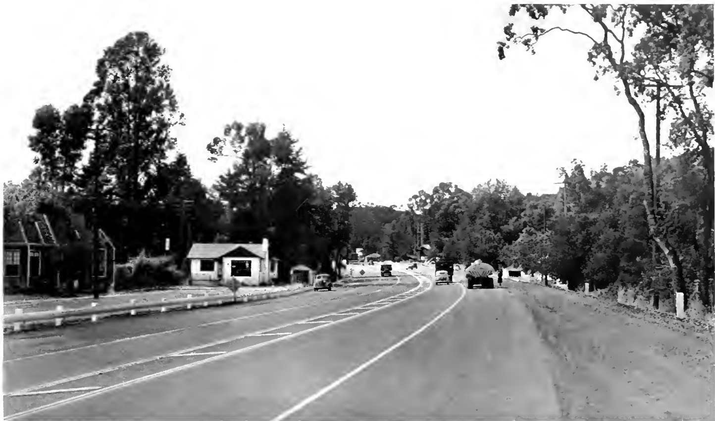
Section of new divided highway north of San Rafael, which will relieve congestion in that city
